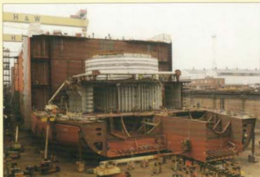
Construction of the Schiehallion FPSO in the Building Dock, clearly showing the lower section of the 14m moonpool. (January 1997)
